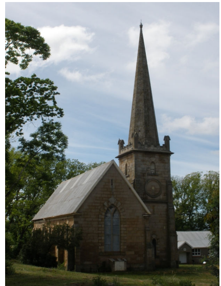
St Andrews Presbyterian Church – waypoint 006
