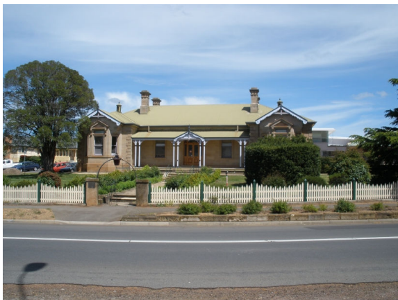
Old Hospital – waypoint 007
